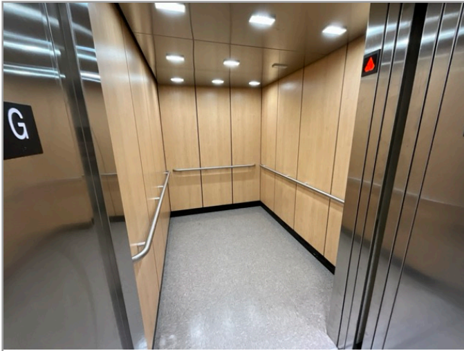
LOBBY LOOKING AT CABS (WITH DOORS OPEN)
