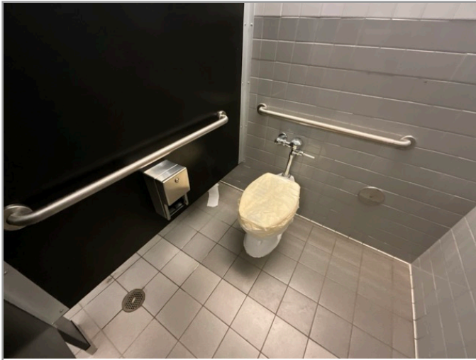
TOILET STALL OVERVIEW
