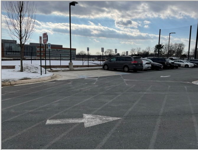
OVERVIEW OF ACCESSIBLE PARKING AREA
